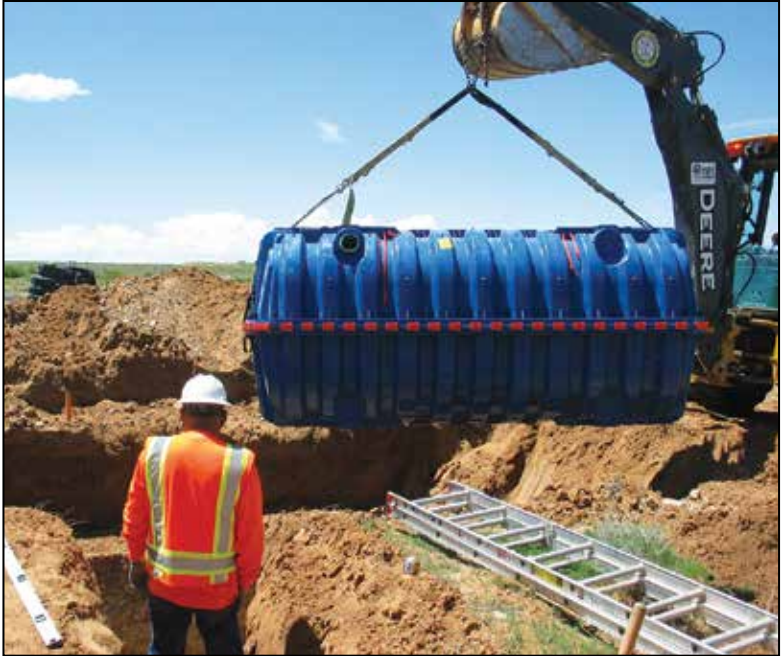
ASDFC worker watches as a septic tank is lowered into the ground to be installed. (Photo Courtesy: IHS Division of Sanitation Facilities Construction)
