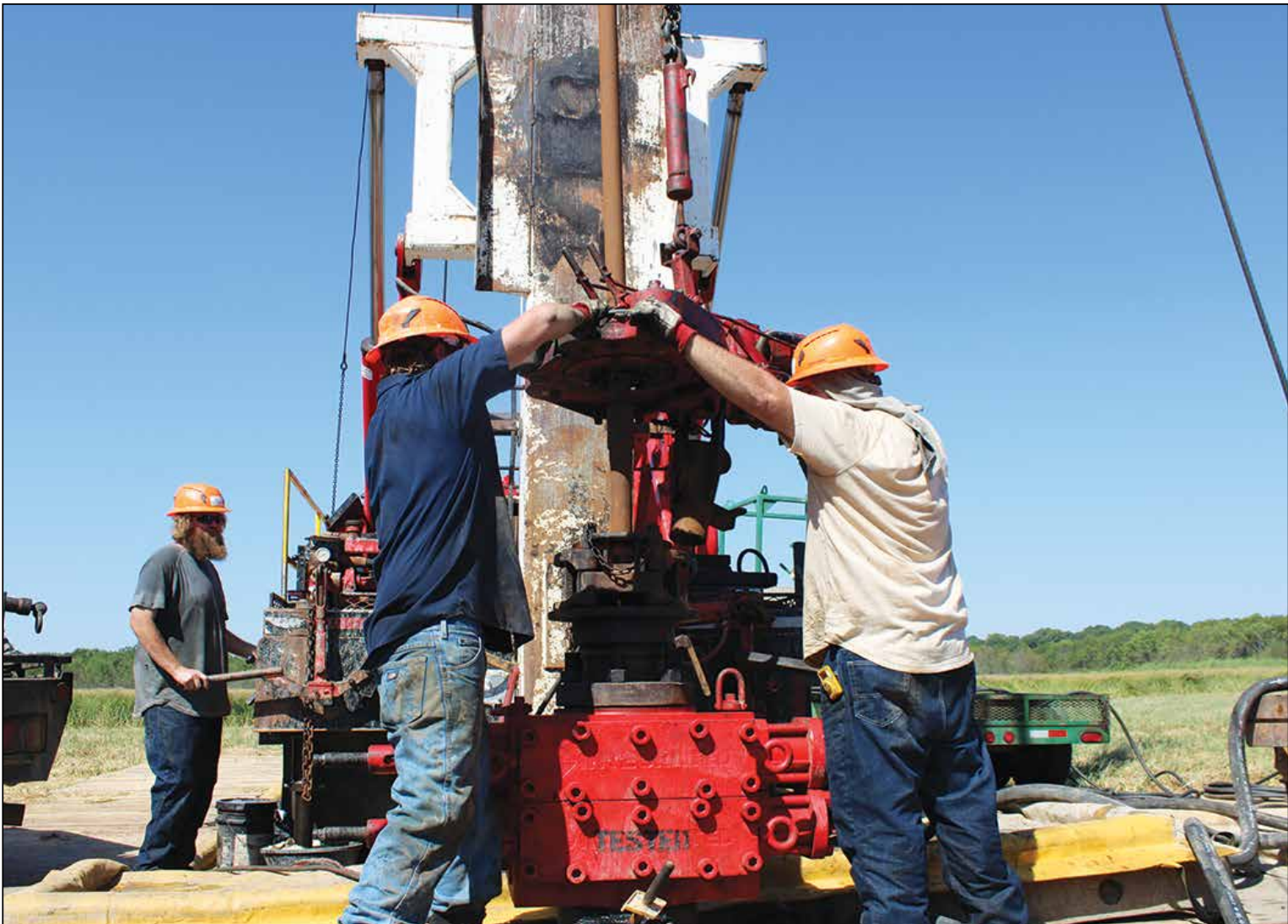
Well Done Foundation contractors are hard at work plugging an orphan well in the Deep Fork Wildlife Refuge. (Braden Harper/MM)
